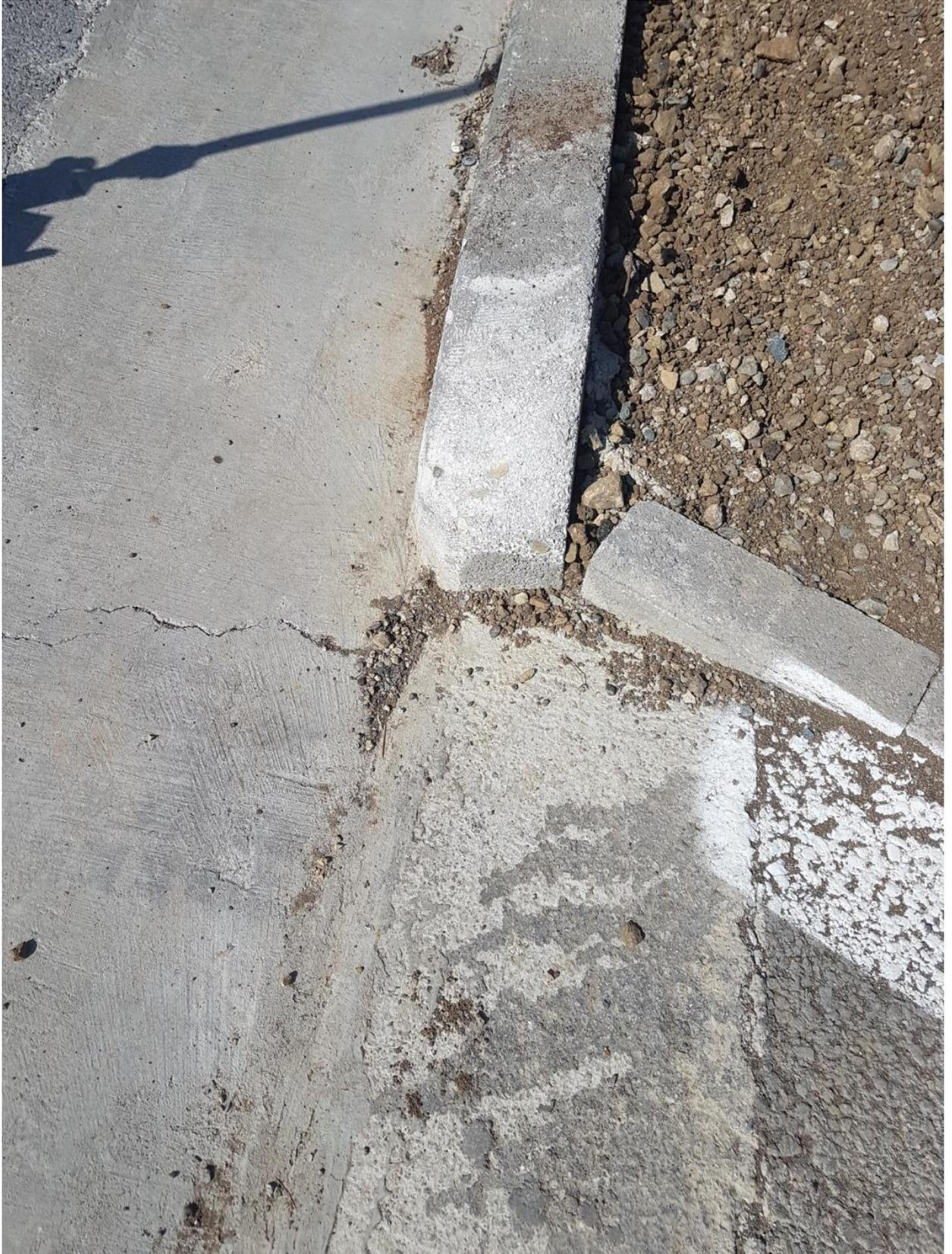
5. Removing the damaged asphalt pavement of the footpath and laying the pavement with new sand asphalt. 15 m<sup>2</sup>.
