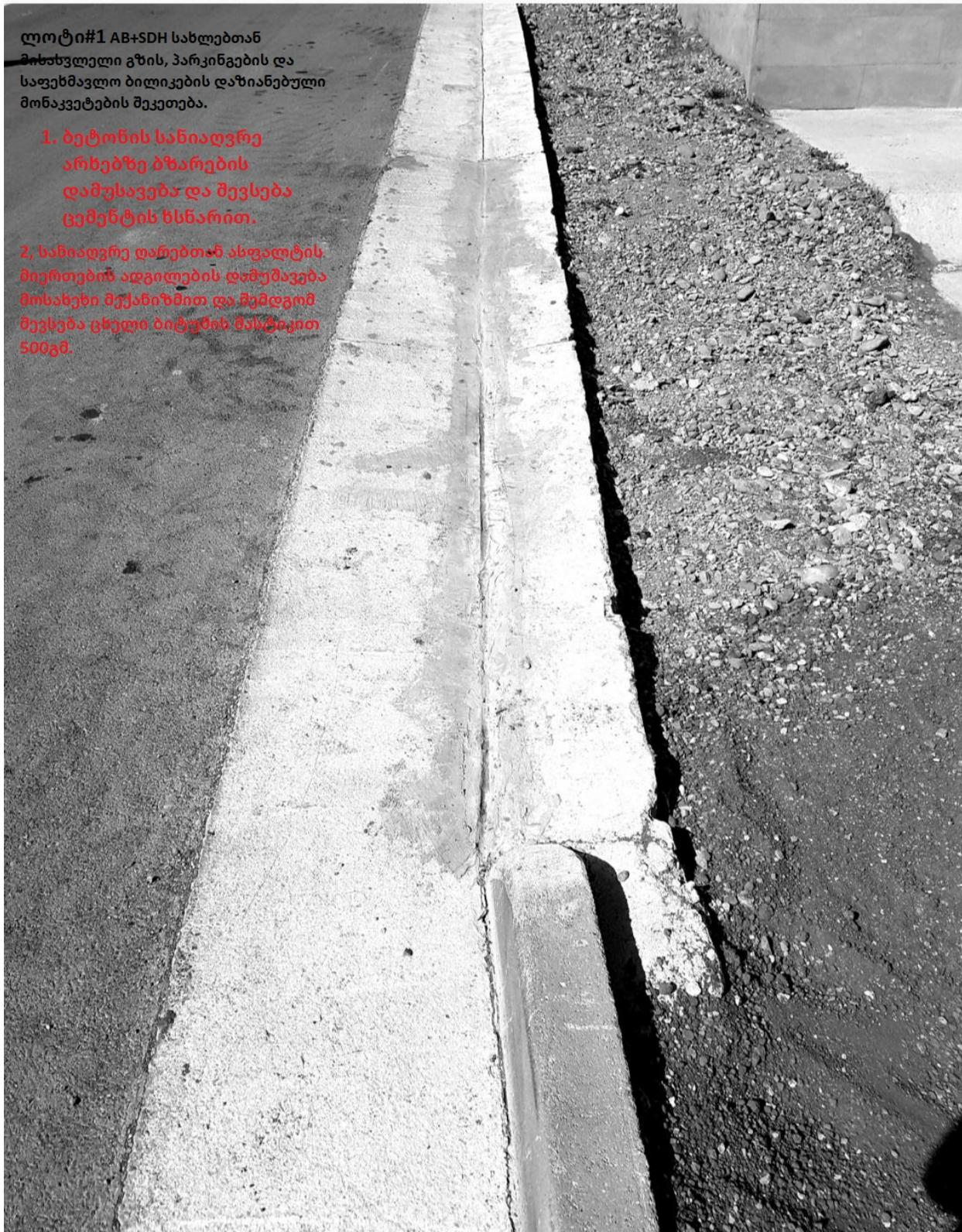
2. Filling the sidewalks joining the sidewalk with a sand-cement mixture.
