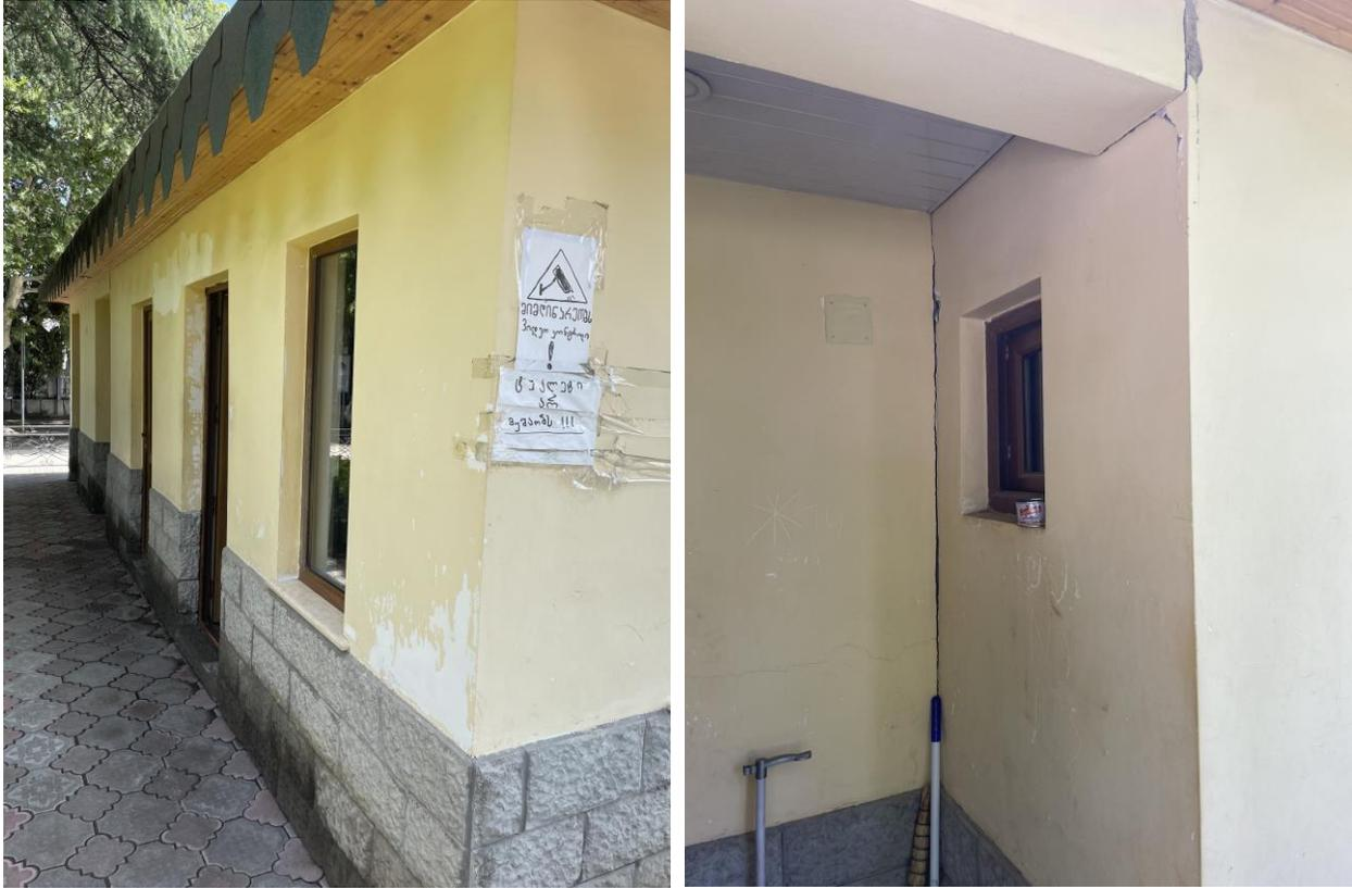
22-Security room indoor painting wall & ceiling. 100 m2. Air conditioner is not working. Brand new one have, but need installation. Spot light need to be changed.
