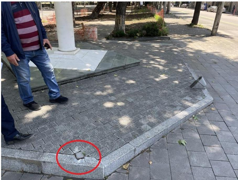
3-Concrete bollars are not fixed on the floor. 4 pieces are moving. 1 piece is not there.
