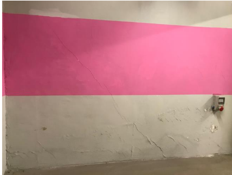
Figure 8 - Cracks in a Wall Perpendicular to the Retaining Wall
