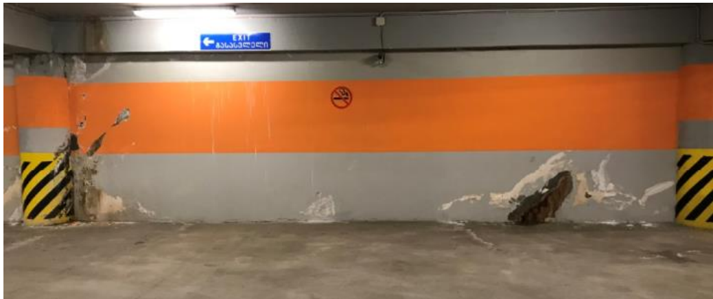
Figure 7 - Cracks in the Retaining Wall
