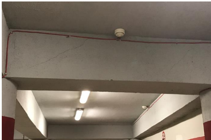
Figure 9 - Cracks in Beams
