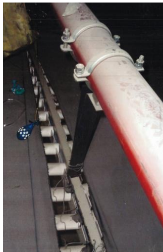
Figure 2 - Hung Facade; The red member is the main structural steel truss.
