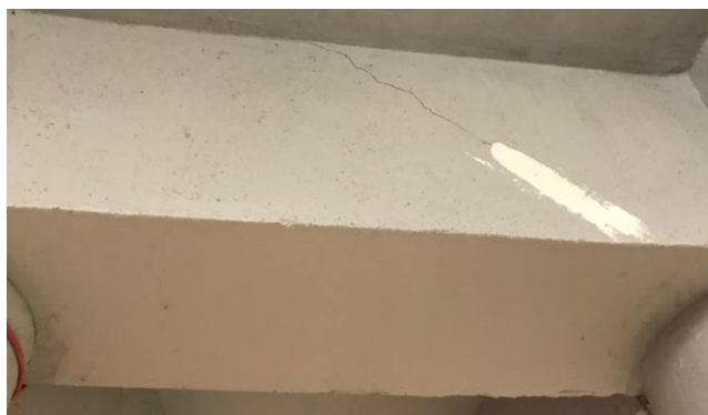
Figure 10 - Repaired Area of a Beam
