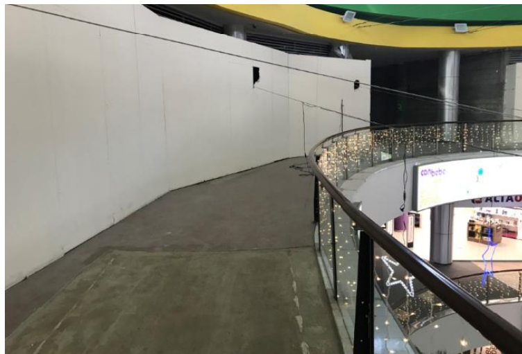
Figure 15 - 3 m Long Cantilever which will not have a back span
