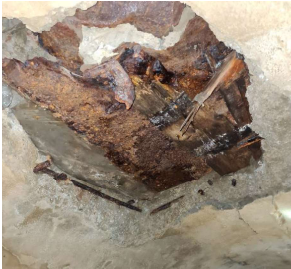
Holes in tunnel bend - pictures N5 and N6
