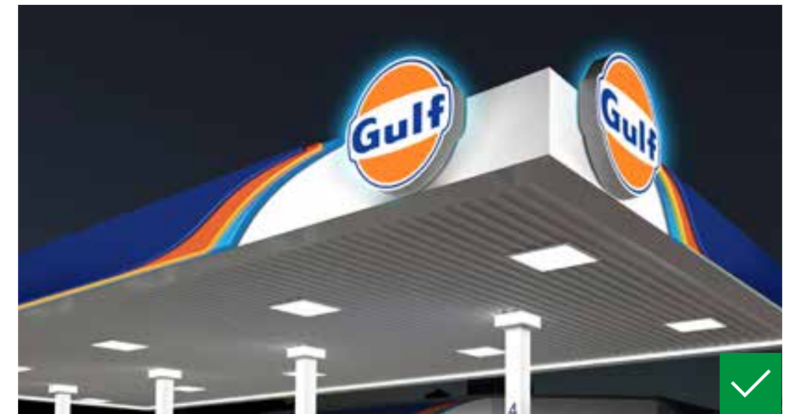
A good example of a canopy – Logos positioned together, but around entrance corners giving maximum standout from every angle.
