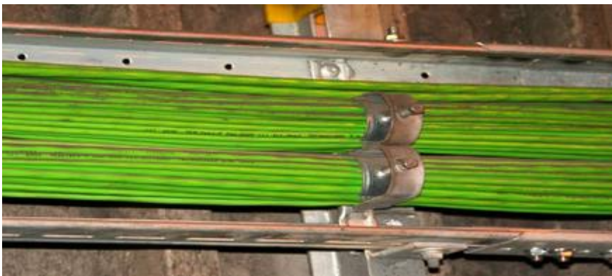
Photo 15: Parallel Cable Installation
